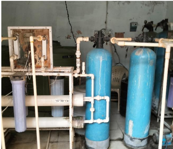
Water RO for water purification
