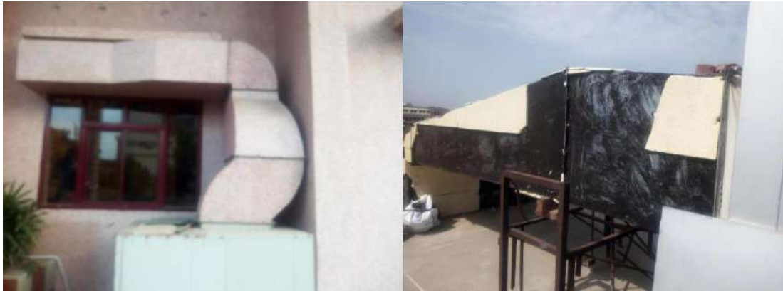
Outside Ducts can be insulated.
